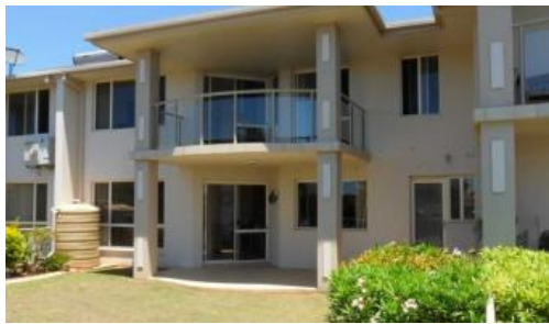
2, 1 Laguna Place, Port Macquarie
