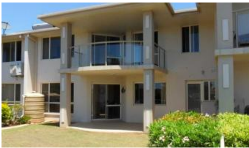
2, 1 Laguna Place, Port Macquarie
