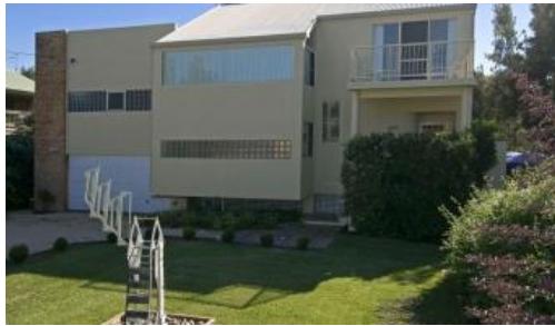
327 Plomer Road, Port Macquarie
