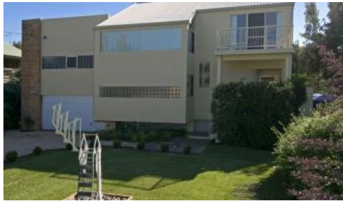
327 Plomer Road, Port Macquarie
