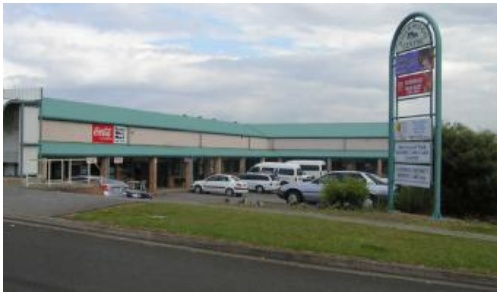
Lot , Lot 31 Friar Close, Port Macquarie
